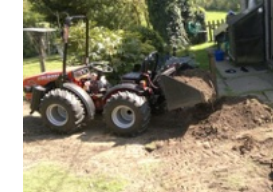
Earth moving on a building site
